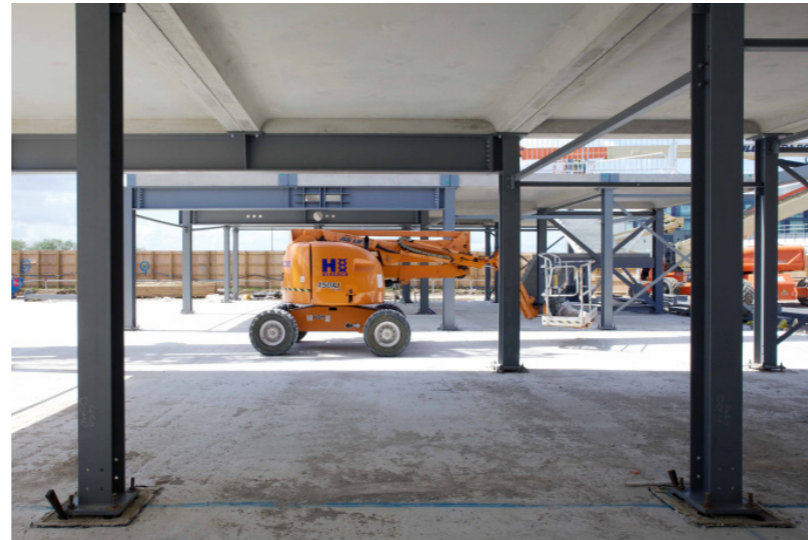
Precast planks partially supported by structural beams.
