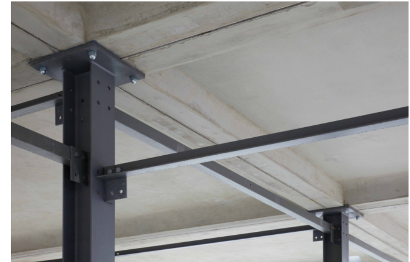
Precast slab to steel column connection detail.
