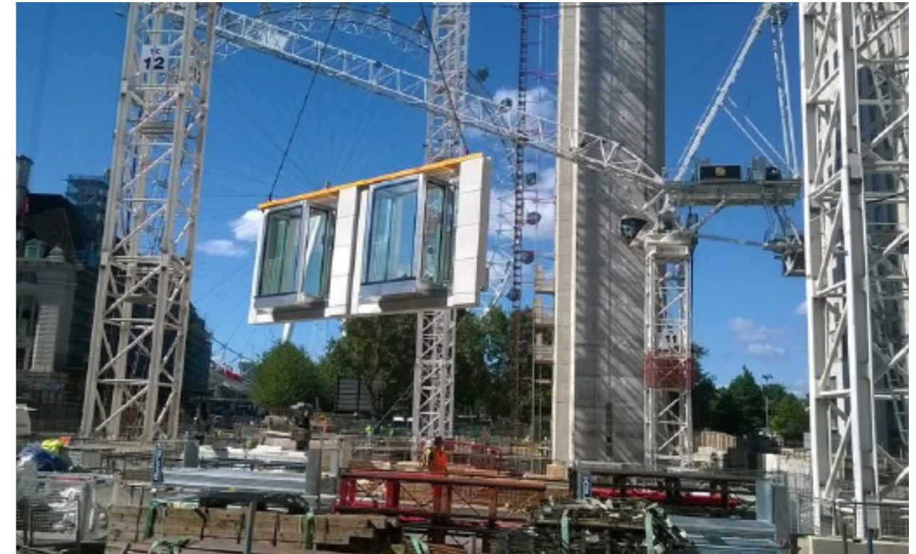
First cladding module lifted on site.
