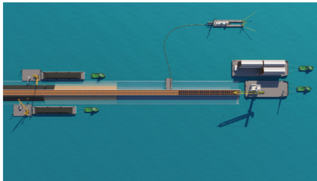
Image showing the linear progression of the prefabricated caisson site assembly stages.
